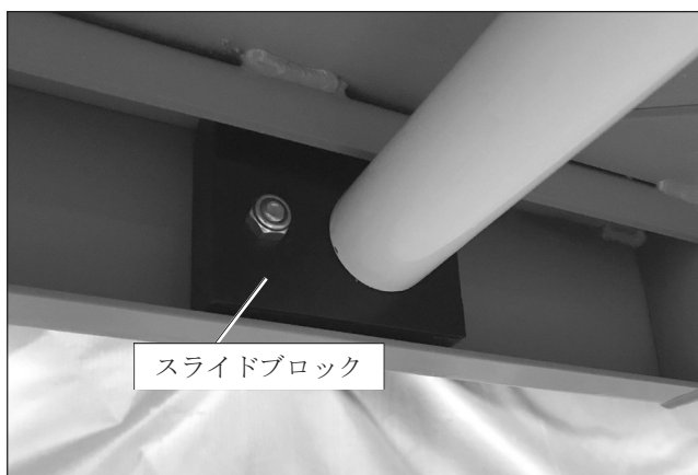
図8.13 - 作業床前部の下側
